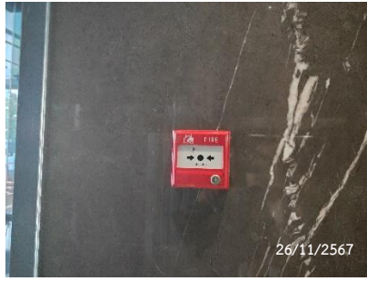
Fire Alarm Manual Station
