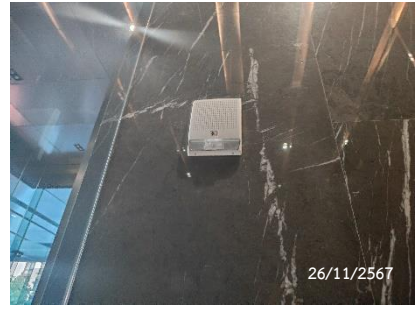
Fire Alarm Horn Strobe
